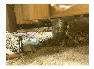
18. The Eastern elevation beneath the bedroom window, there is a garden mulch and open porous garden beds hard up against the external wall of the home.
