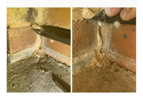
6. The entire bottom brick mortar is deteriorating.
