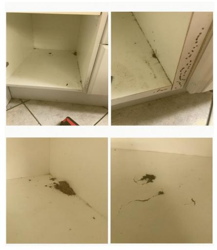
57. Within the carcass located to the right side of the fridge and left side of the pot drawers, the bottom shelf of the carcass has been completely eaten out by termites.
