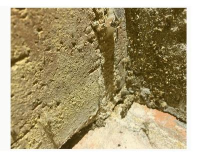
5. Second possible termite entry point into the garage was within the third brick pillar along the left side of the garage approx. 5 m from the garage door.
