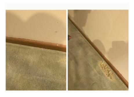
48. In the image above there is a second mud tunnel seen on top of the timber skirting board below the staircase.
